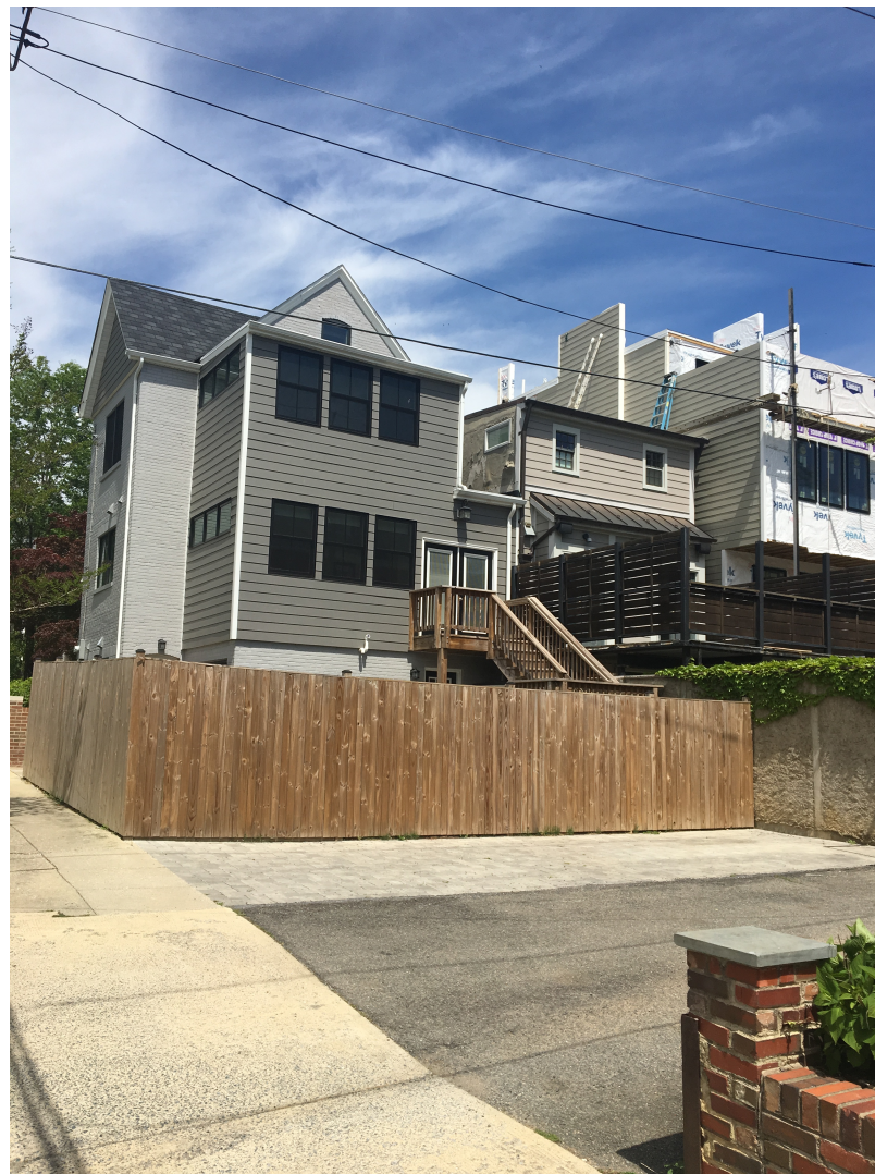
View Public Alley intersecting 38th Street NW
